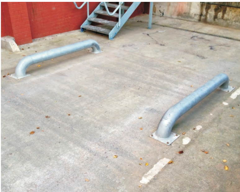
Galvanised finish wheel guide on loading bay
