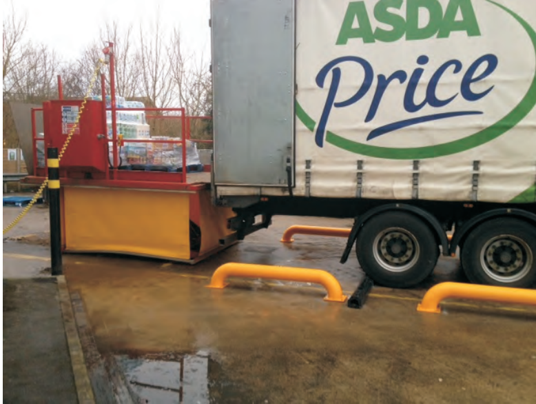
Wheel guide situated on ASDA warehouse
